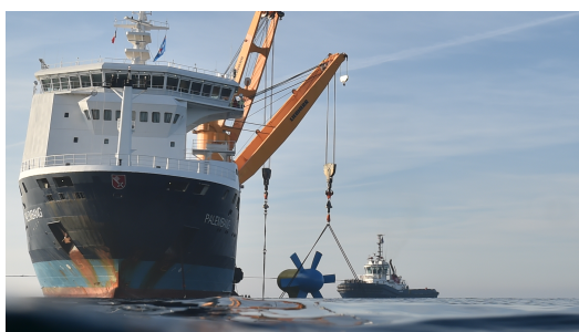
A SABELLA turbine being lowered into the sea
